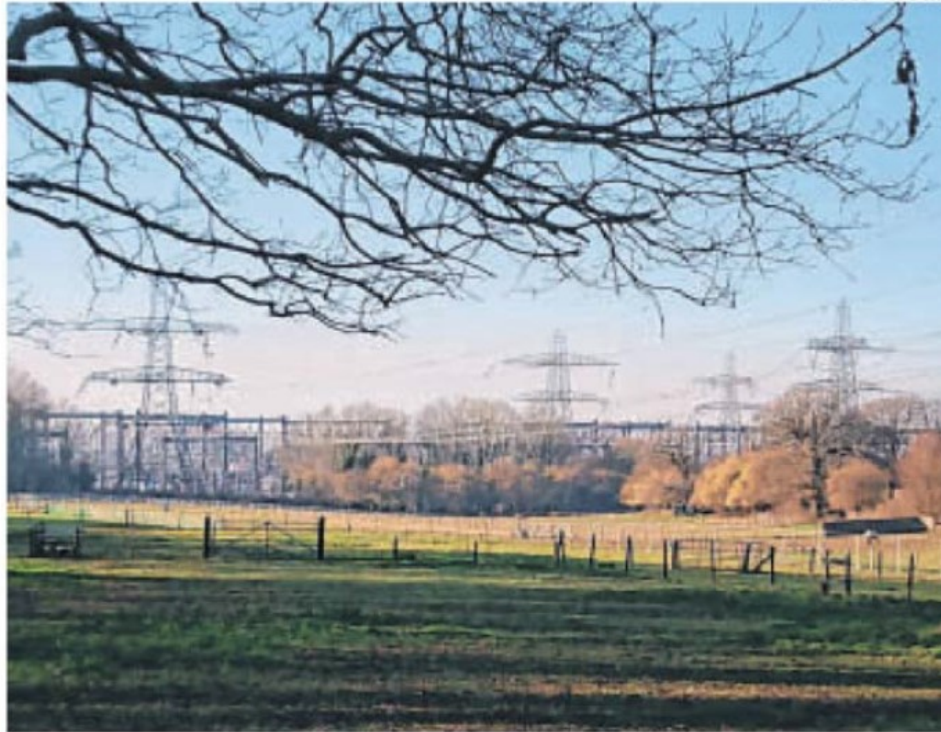
Land west of the Lovedean substation has been earmarked by Aquind for a converter station.
