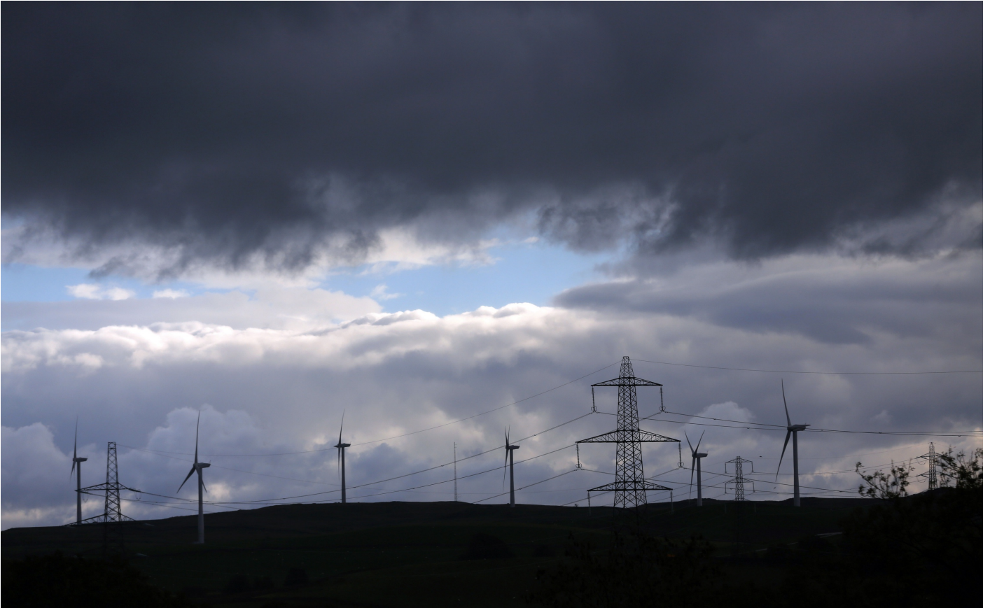
Wind turbines stand on the horizon near a National Grid Plc electricity pylons in Kendal, U.K. Photographer: Paul Thomas/Bloomberg
